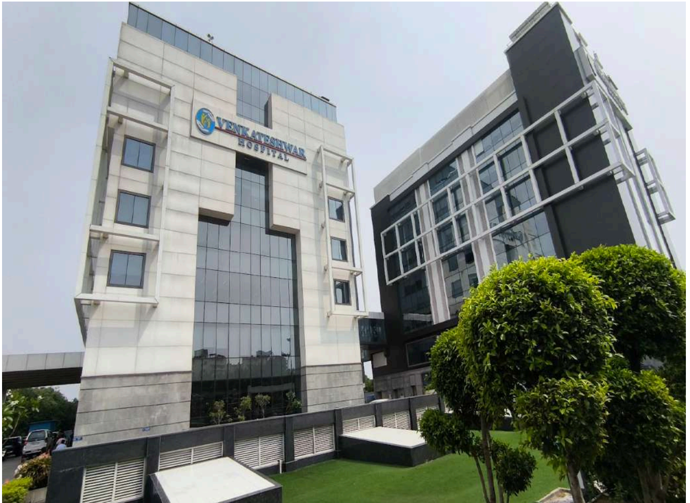
PHOTOGRAPHS OF OPERATIONAL BUILDING
