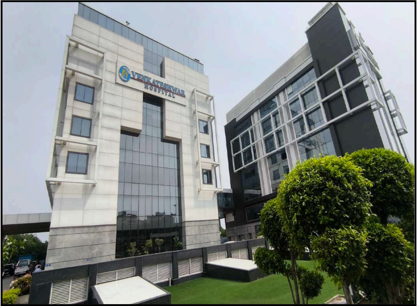
PHOTOGRAPHS OF OPERATIONAL BUILDING
